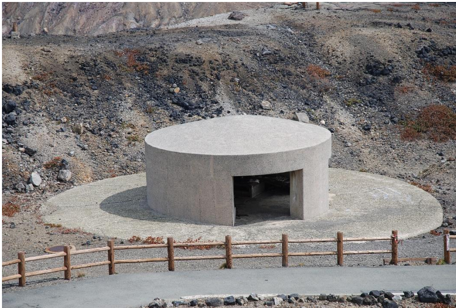
Figure 3: Concrete shelters used in Japan next to an active crater. These shelters are built from reinforced concrete and can hold around 50 people
